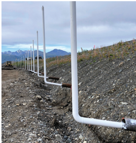
Figure 5: Final thermosyphon riser piping before installation of radiators and backfill
