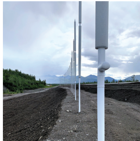
Figure 6: Completed thermosyphons with vertical radiators installed and backfill complete
